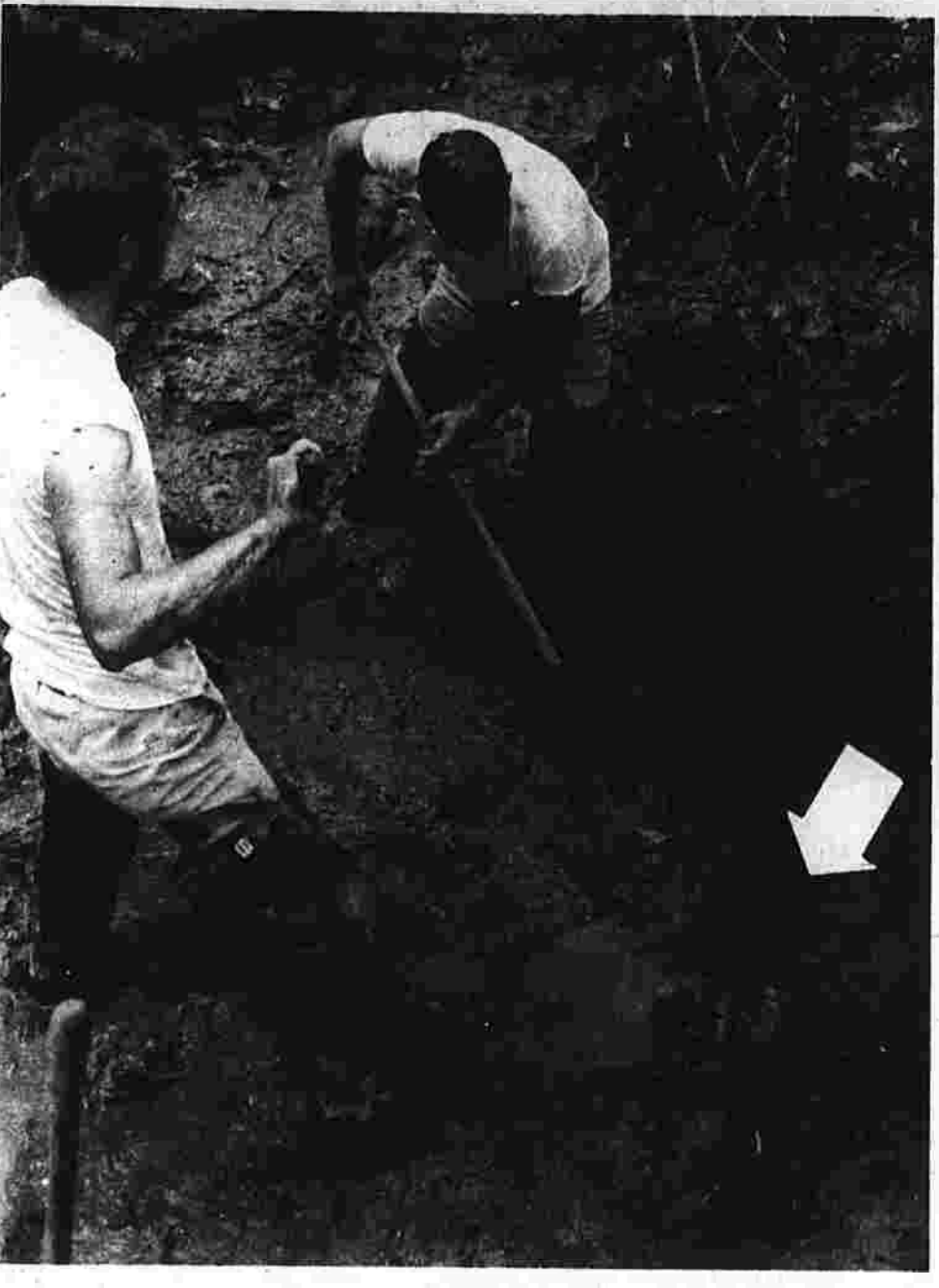
Town of Manchester Public Works personnel work to uncover the ruptured wooden pipeline, indicated by the arrow. The pipe line was shattered Wednesday morning when a bulldozer ran over a boulder, forcing it down through four feet of soft ground, smashing the pipe. The metal spiral visible in the mire was a part of the wooden pipeline, which was made up of planks, wrapped tightly with wires. By about 3 p.m. the repair crew had the damaged section of pipeline uncovered. (Herald photo by Knapp)
