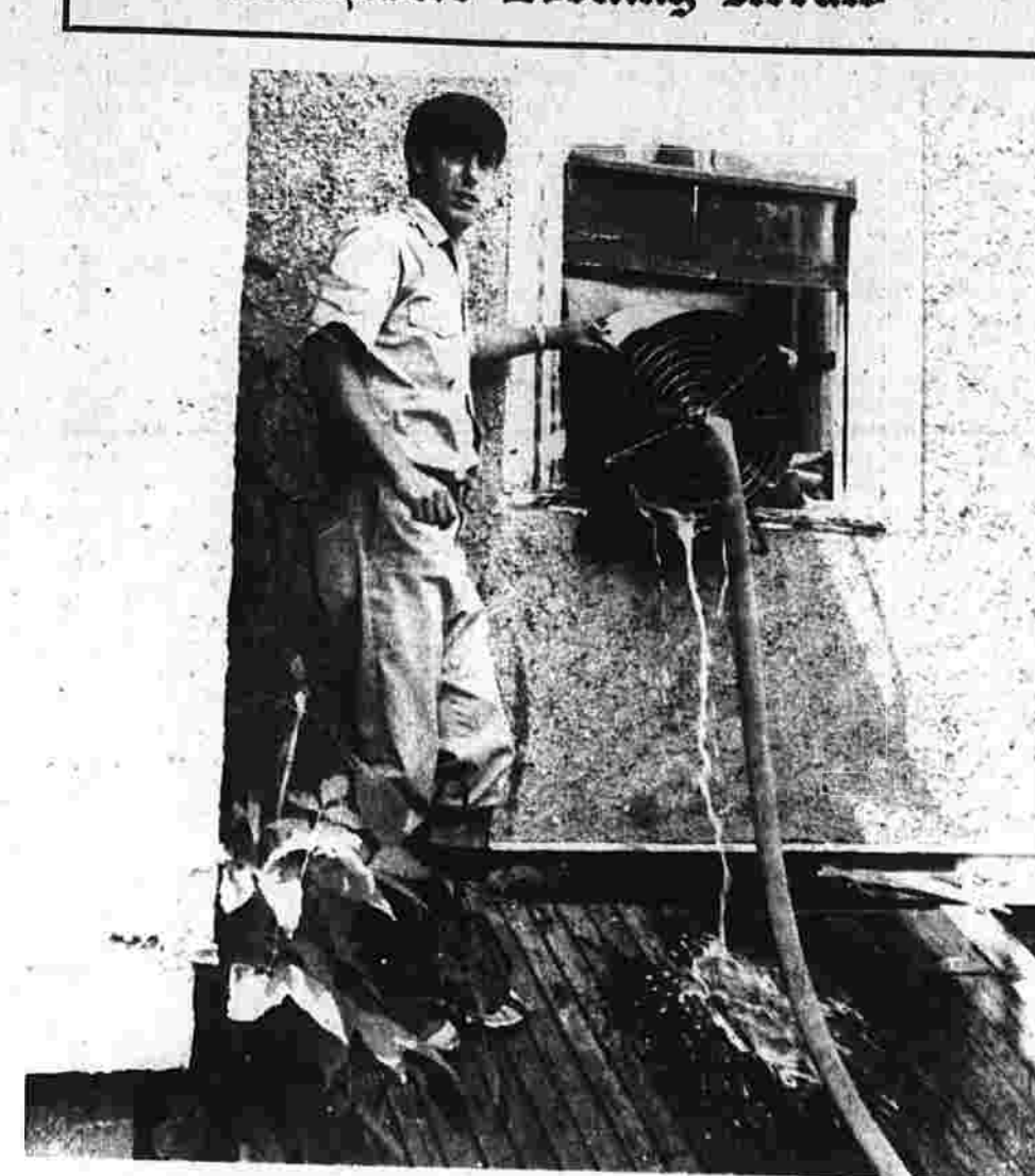
Fireman John Hughes of 27 Dudley St. mans a foam disperser unit as he fills the house with foam. The unit is fed through a 1 1/2-inch line from a pump truck. Firemen say that an average size house can be filled with foam in approximately five minutes using this method.
