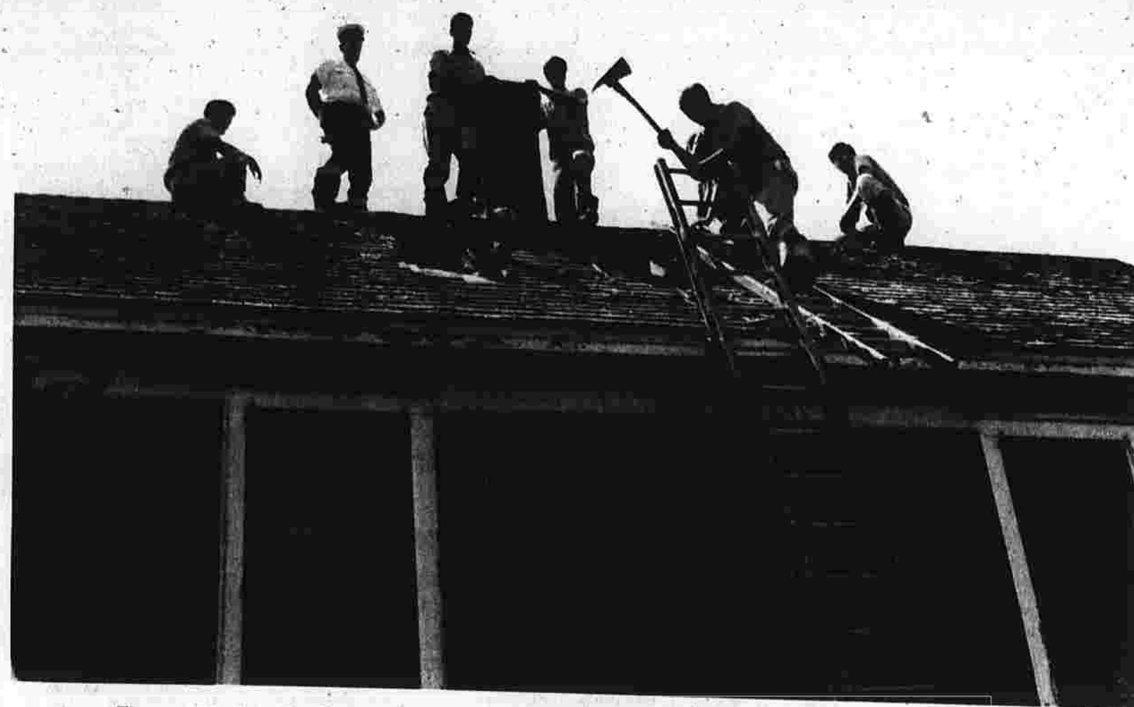
Firemen of the Town Fire-Department practice chopping ventilation holes in the roof of a building at 353 Main St.
